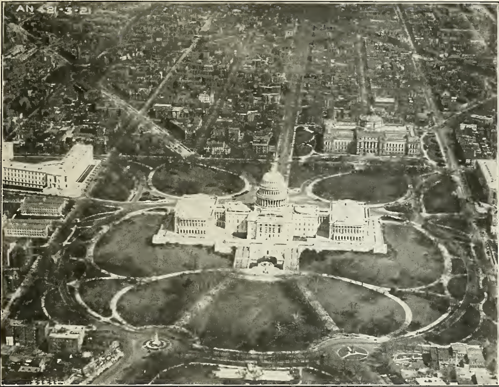
Only from the air can this extraordinary detailed geometric planning be seen. Grouped about the Capitol may be seen in the front the Grant Memorial; on the extreme right part of the Representatives' Office Building; the Congressional Library, and at the left the Senate Office Building. The Capitol itself is one of the finest examples of balanced architectural planning in the world.
